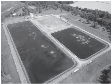
Lagoon #3; sludge removed, before new liner
