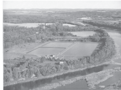
Wastewater treatment plant located on the Grimes Road
