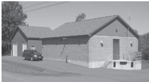
Water treatment plant located on the River Road
